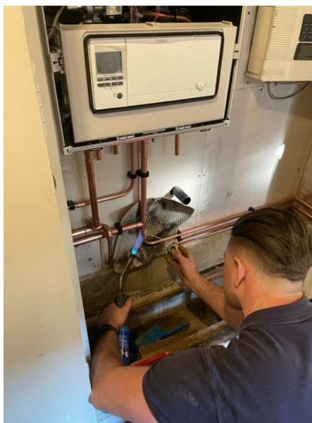
Soldering copper pipework under a boiler I have just installed in the Amen Court.
